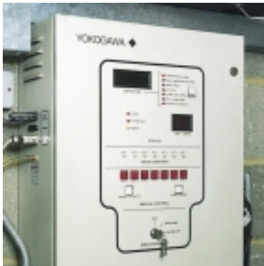
Refrigerant gas leak detection system
