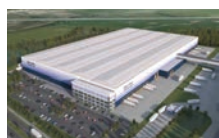
A new warehouse will be built alongside our current one at Magna Park to support the ongoing online growth
