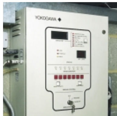
Refrigerant gas leak detection system
