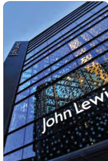
John Lewis Cardiff gets 100% of its electricity from the incineration of demolition waste.
